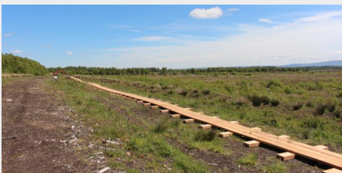
Simple floating boardwalk installed at Bolton Fell Moss © Natural England
